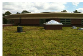
Ballast system Extensive roof
