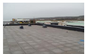
Ballast system 50mm concrete slabs
