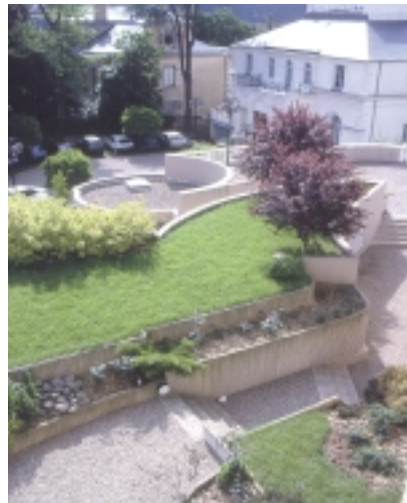
Right: Intensive roof garden over housing. Range of both hard and soft surfaces.
