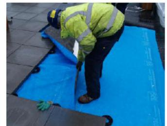
**2 - Ensure joints in the tape overlap. Pull back the top protective layer of the tape.**
