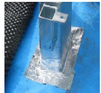
**3 - Pull and overlap the joints of the membrane to provide a minimum 150mm lap.**
