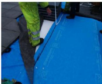
**5 - Apply sealing tape to upstand, using a neoprene roller to apply pressure. Pull away protective cover and bring Hydroshield membrane up and into contact. Finish the detail by using the roller to complete the seal.**
