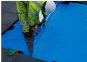
**4 - Ensure a full seal at all membrane laps and joints with pressure. Install ballast immediately.**
