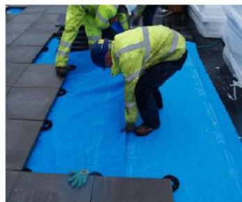
**6 - Trim Hydroshield membrane neatly to detail. Apply Stickband forming a continuous seal around edges, applying pressure with roller. Stickband is used to seal the edges of the Hydroshield membrane to the waterproofing surface at penetrations and outlets.**
