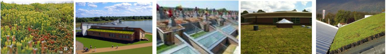
Maintenance, conducted by qualified personnel, will ensure the initial establishment and continued health of the green roof system. It is strongly recommended that the installing contractor remains responsible for the maintenance of the green roof during this establishment stage (between 12 - 15 months) and prior to the assignation of maintenance duties to the building owner's representative. Maintenance contractors with specialist training in green roof care should be used where possible.
